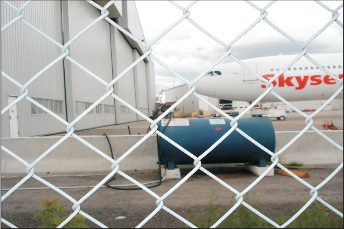
Photograph 3: View of an approximately 500-gallon diesel AST, looking north
