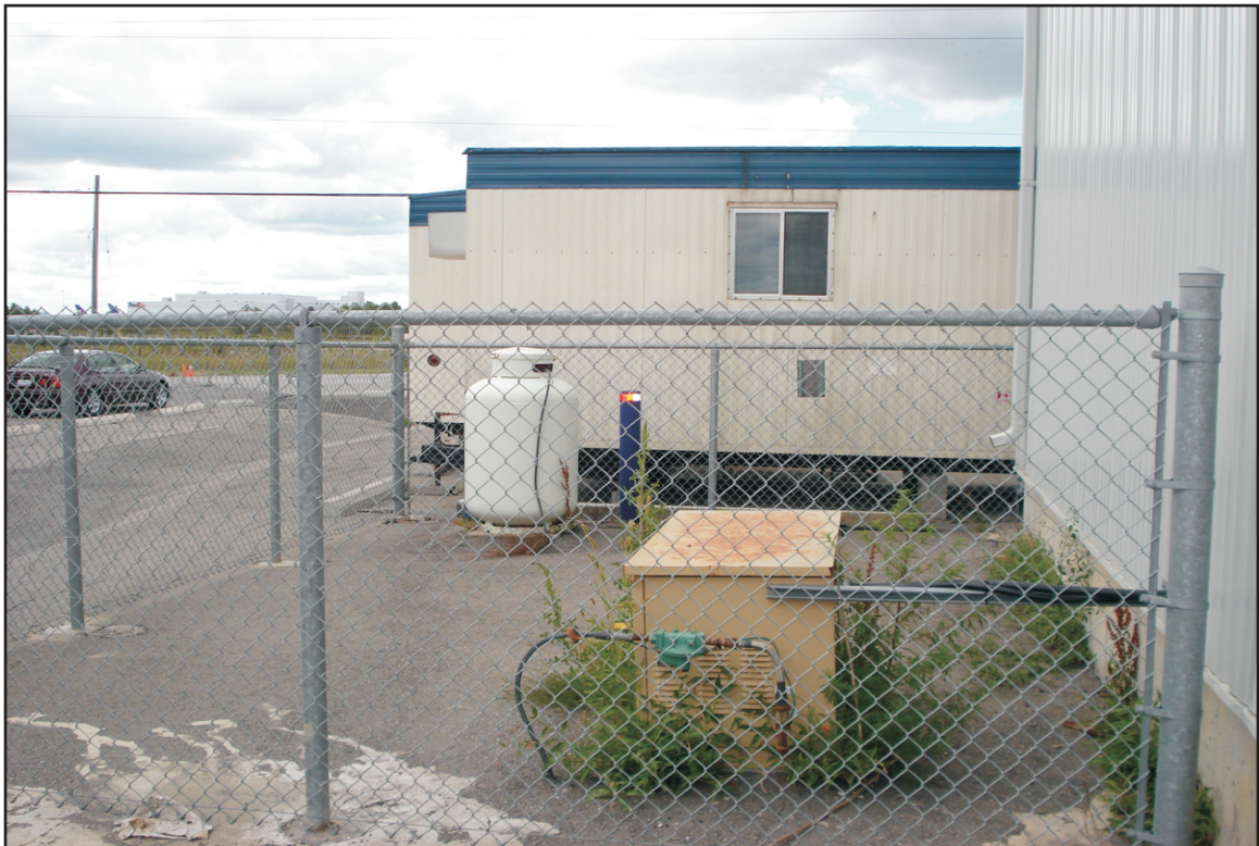
Photograph 2: View of the Propane-fired emergency generator and propane tank looking west.
