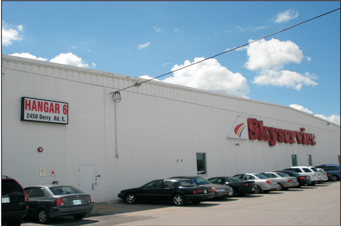
Photograph 1: View of the Site, looking south.
